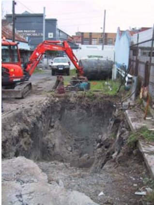
Commencement of Works
